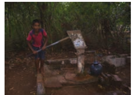
Non-piped sources do not provide reliable supply of water throughout year
